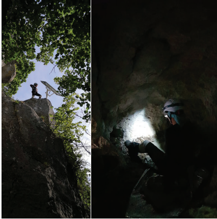
Installation of a seismic station (TEMA, Slovakia)
